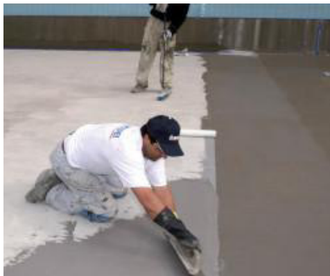
Waterproofing a swimming pool with Mapelastic Zero
