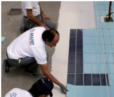
Application of ceramic coating on Mapelastic Zero
