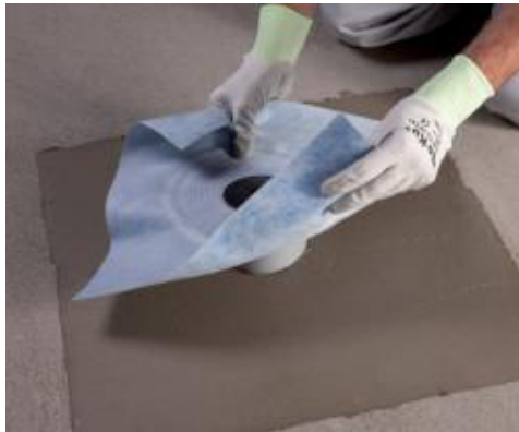
Application of Drain Vertical on Mapelastic Zero
