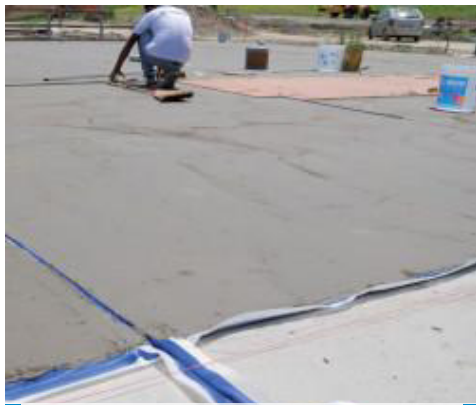
Waterproofing screeds with Mapelastic Zero and Mapeband
