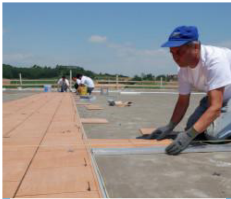
Laying ceramic tiles with Kerabond + Isolastic
