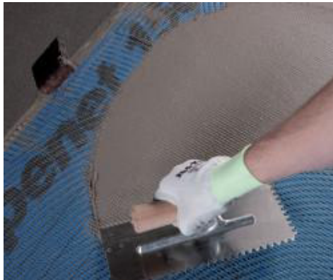
Application of Mapelastic Zero on Mapenet 150
